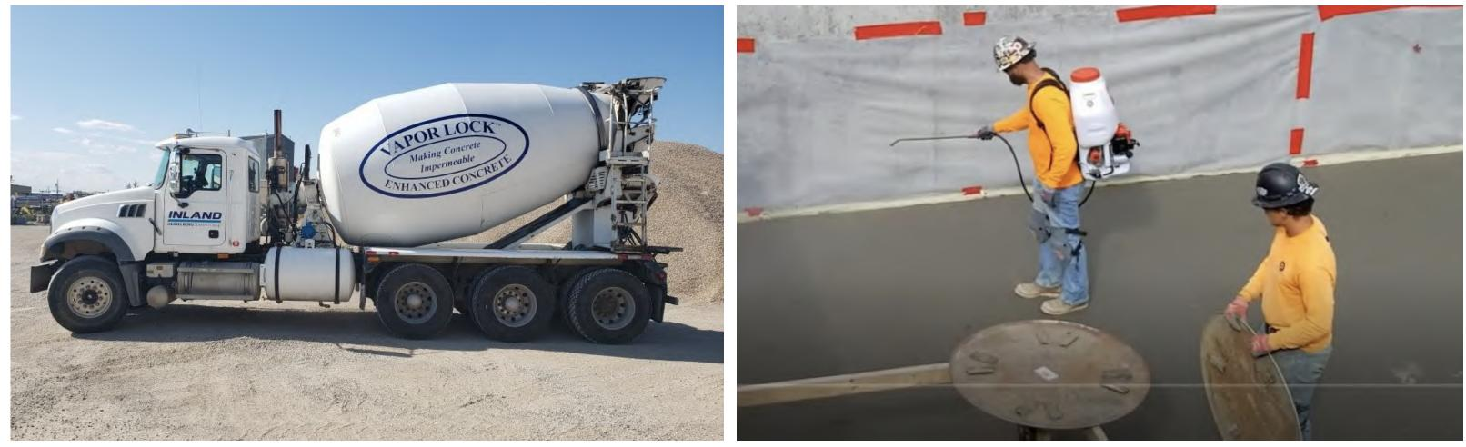
With an extensive track record of proven performance, **Vapor Lock** begins the densification process inside the concrete truck reacting with the calcium hydroxide formed by Portland cement. This virtually eliminates the porosity of the concrete, providing a platform to maximize densification. **Vapor Lock 1** is applied to the surface during the troweling/panning process, furthering densification to an extreme degree.
